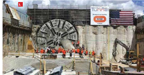
1. Extensive works were carried out to ensure the project remained on track (image courtesy of Daniel Azoulay) 2. Safety measures were implemented to protect construction personnel from the live traffic running alongside the project (image courtesy of Florida Department of Transportation) 3. The route of the Port of Miami Tunnel runs through soft ground conditions and was driven using a specially configured TBM (image courtesy of Daniel Azoulay) 4. Construction operations were extensive (image courtesy of Florida Department of Transportation) 5. The Port of Miami Tunnel has been constructed despite major challenges, both technically and financially (image courtesy of Daniel Azoulay) 6. Free flow tolling technology ensures optimum capacity (image courtesy of Florida Department of Transportation)
